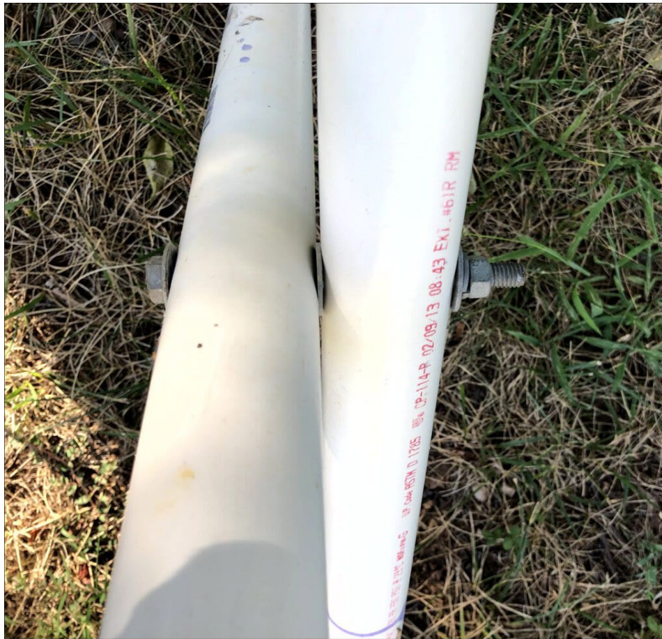
Figure 3 - Detail of Pivot Bolts Through the PVC Pipe
