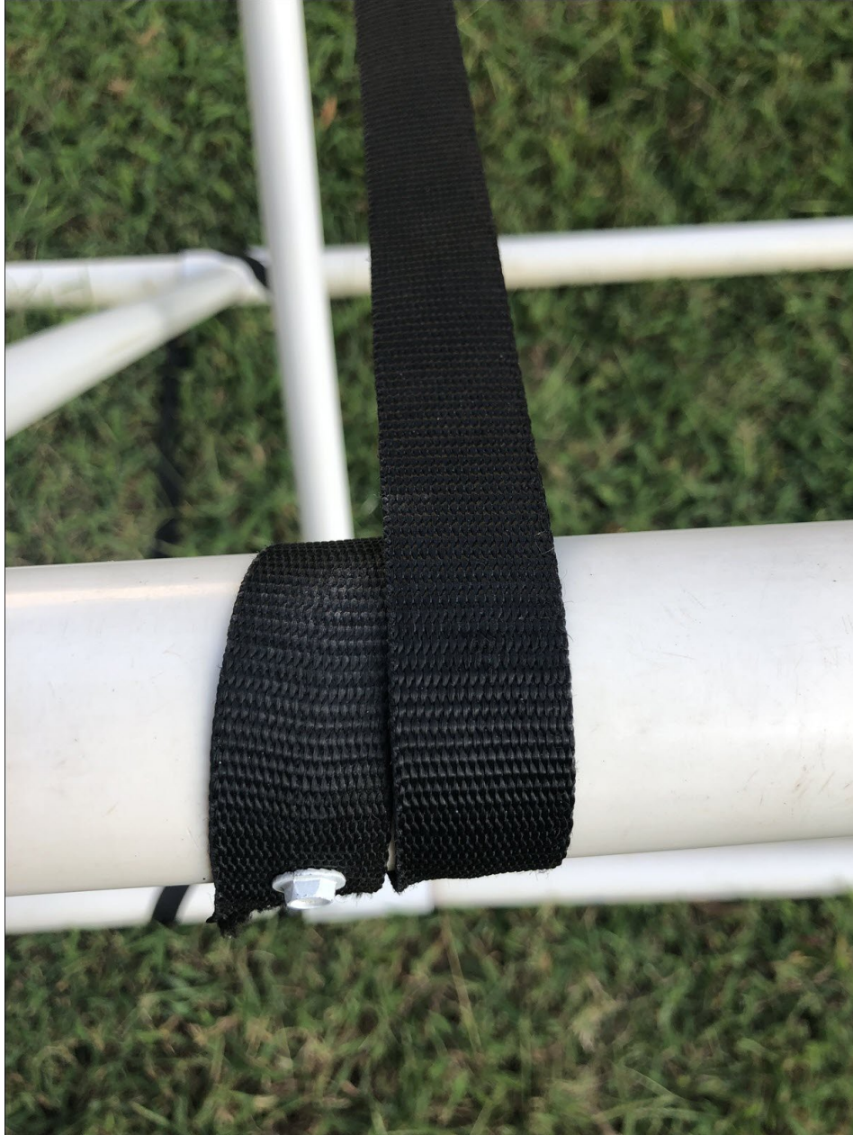
Figure 12 - Detail of Nylon Strap Installation
