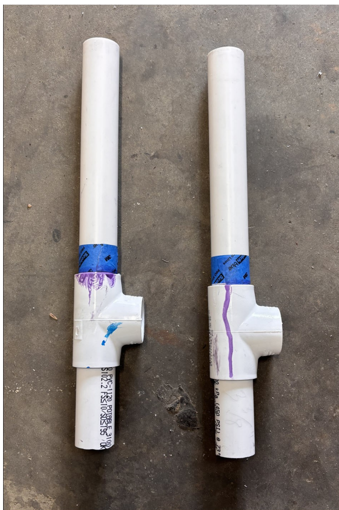
Illustration 7: Use Painters Tape to Mark Alignment
